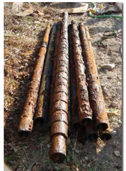
Pump turbine shafts after removal.
