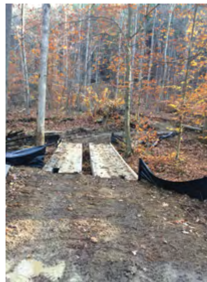
Excavators were mobilized for the construction of temporary access roads and stream crossings. When work was completed, the area was reclaimed back to its original contour.
