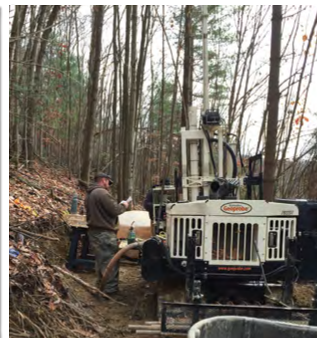
Logging one of the 64 borings completed at the site.
