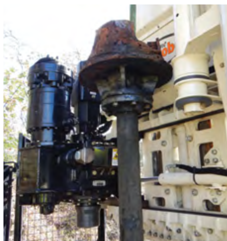
3230DT pulling well shaft.
