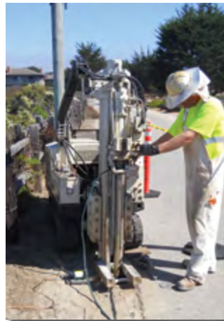
One MiHpt location (MIP-14) was within the active Monterey Bay Coastal Recreational Trail. Jeff Edmonds, with ECA, operates a Geoprobe® 54LT at this location in order to minimize the impact to the trail and its users.
