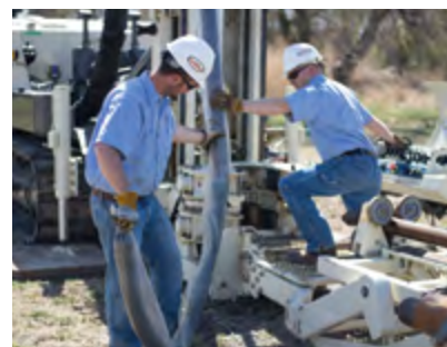
(right) A wireline overshot is released from the modular weight assembly during the sample collection process. The use of the winchline for retrieving sample sheaths reduces 'trip in' and 'trip out' times significantly.
