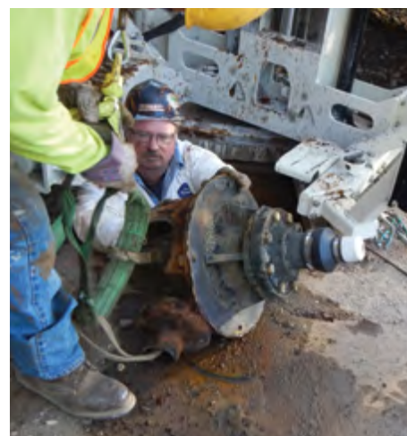
Rigging top of discharge head.
