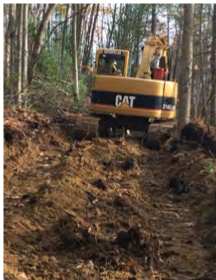
Excavators were mobilized for the construction of temporary access roads and stream crossings. When work was completed, the area was reclaimed back to its original contour.
