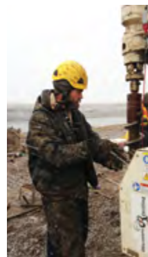
Derek Dell, Driller for Discovery Drilling, advances 3.25-in. hollow stem augers using the GA2500 auger on the 6712DT.
