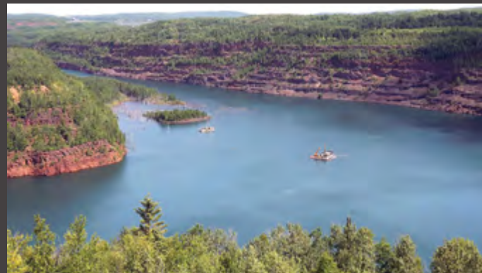
Aerial view of Rouchleau Pit in Virginia, MN, proposed site of a new bridge carrying US Highway 53 for rerouting the highway. IDEA Drilling used an 8140LS Sonic rig (on upper barge) to collect core samples. The 8140LS, because of its compact footprint, was able to work from a smaller barge than another rig used onsite. (online News Tribune file photo)
