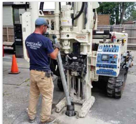
(above and right) A cathodic anode is installed through the inside diameter of DT60 casing at a UST site. What was thought to be a single-day project with no return business for Horizon Construction and Exploration, has developed into a weekly cathodic anode installation job at various sites in the midwest.
