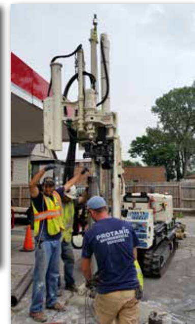
(above and right) A cathodic anode is installed through the inside diameter of DT60 casing at a UST site. What was thought to be a single-day project with no return business for Horizon Construction and Exploration, has developed into a weekly cathodic anode installation job at various sites in the midwest.
