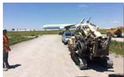
A 7822DT completes monitoring well installation airside at Pearson International Airport.
