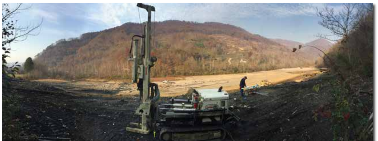
Confirmatory UST sampling for petroleum hydrocarbons with the 7822DT overlooking Black Mountain in Kentucky (Kentucky's highest peak at 4,400 ft.) near the Virginia border.
