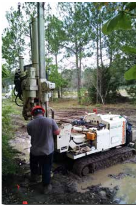
(above and below) Drew Small with TRS contacted Geo Lab to assist with ERH electrode installation at an active manufacturing facility near Murphy, NC. For this most recent phase, Geo Lab installed supplemental electrodes, as well as obtained continuous soil samples with soil temperatures around 200 degrees F. A 7822DT pulled the continuous hot soil samples, from 100 ft. bgs, by advancing a Macro-Core® sampler with stainless steel liners to withstand the heat. Following the sampling, Geo Lab installed multiple electrodes to greater than 100 ft. using hollow stem augers, requiring very careful handling of the steaming mud. After completion, Drew Small said that in the early stages of the project he had his doubts as to whether the scope of work could be completed. "I was impressed with the capability of the rig and your guys during this install," he said. "I wasn't sure it was possible."
