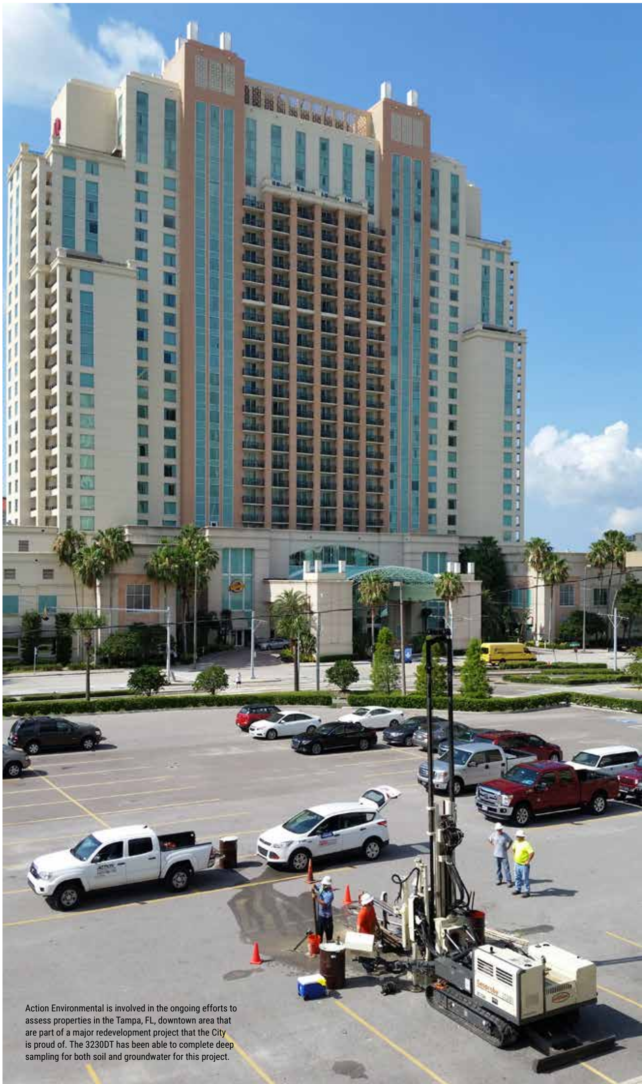
Action Environmental used their 3230DT to complete soil and groundwater sampling needed to assess the properties in downtown Tampa that were planned for future development.
