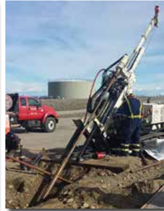
Air rotary casing advancement at a 45 degree angle with the 7822DT.
