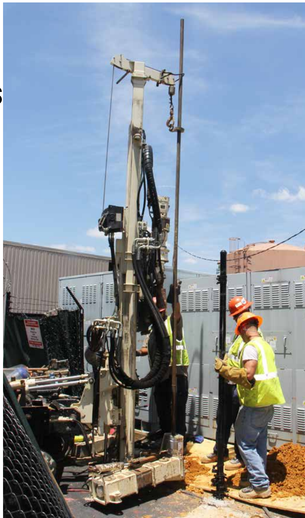
(above and below) Drew Small with TRS contacted Geo Lab to assist with ERH electrode installation at an active manufacturing facility near Murphy, NC. For this most recent phase, Geo Lab installed supplemental electrodes, as well as obtained continuous soil samples with soil temperatures around 200 degrees F. A 7822DT pulled the continuous hot soil samples, from 100 ft. bgs, by advancing a Macro-Core® sampler with stainless steel liners to withstand the heat. Following the sampling, Geo Lab installed multiple electrodes to greater than 100 ft. using hollow stem augers, requiring very careful handling of the steaming mud. After completion, Drew Small said that in the early stages of the project he had his doubts as to whether the scope of work could be completed. "I was impressed with the capability of the rig and your guys during this install," he said. "I wasn't sure it was possible."
