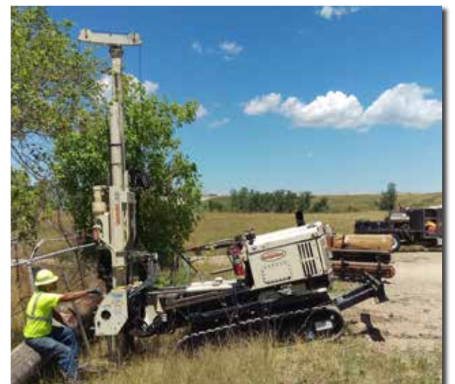
Tom Ulrich, Driller/Crewchief, is caught sitting down on the job while taking soil samples in an old landfill to help determine the extent of the contamination cell.
