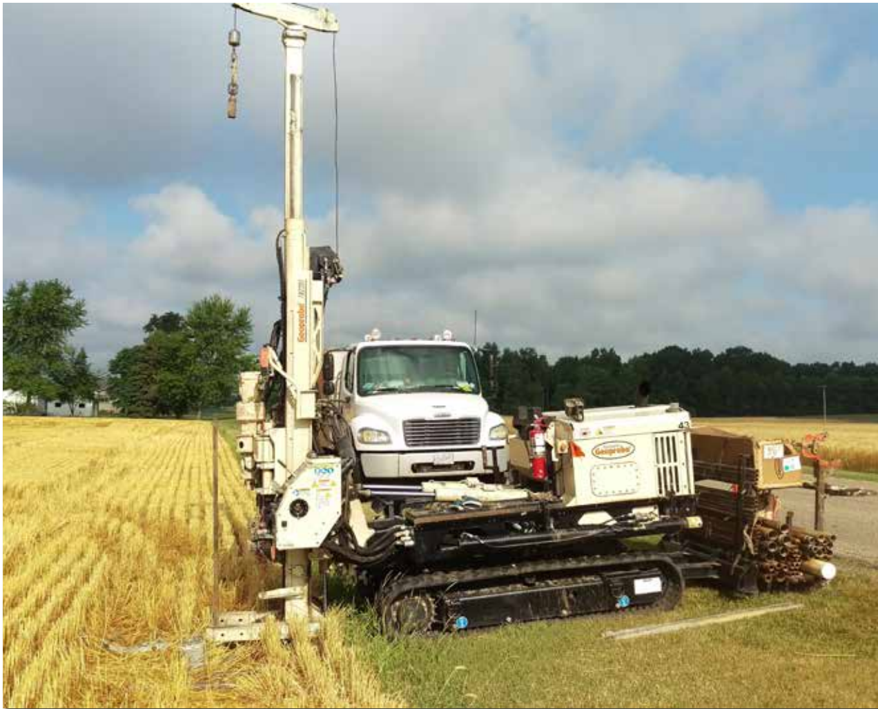
Stearns Drilling uses their 7822DT to work on a bedrock study for the Michigan Division of the U.S. Geological Society in conjunction with Western Michigan University.
