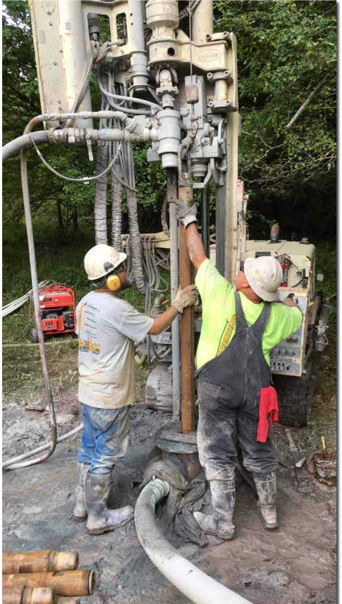
Connor Neely, Driller (left), and Chris Chronister, Eichelberger Field Superintendent, add a drill rod during the 5-in. air percussion drilling.
