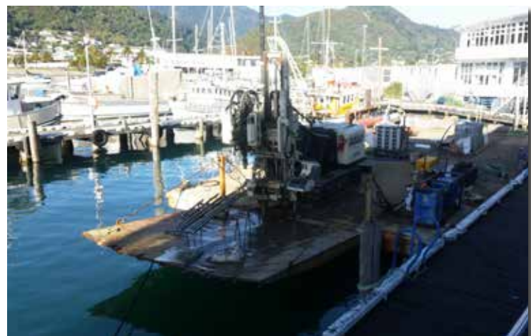
McMillan Drilling's sonic rigs have found projects in various environments, both on land and off shore.
