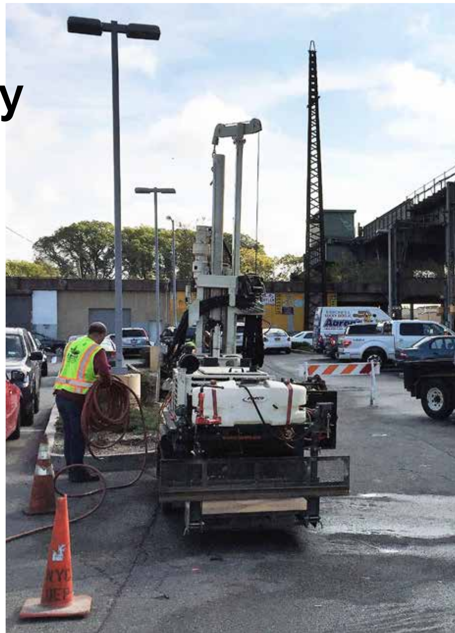
Because of a persistent and ongoing historical contamination, Brian McCabe and Steve Bitetto (in front of rig), with EPhase 2, install the new EKF remediation technology at a site in Queens, NY.
