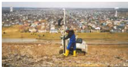
Using a 54DT and Macro-Core® sampler to collect soil cores on top of a landfill to measure clay/soil cap thickness.
