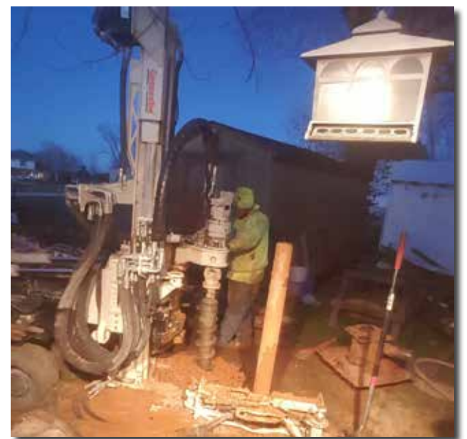
Soil sampling with the 7822DT to bedrock at 45 feet, augering to bedrock at 45 feet, then air rotary to 57 feet to set a 2-in. monitoring well. All in a day's work for RAZEK!
