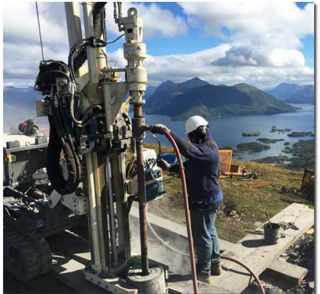
Soni Makihele, Driller, advances air rotary tooling through bedrock on a remote mountain top. The 6712DT was mobilized via helicopter long line.
