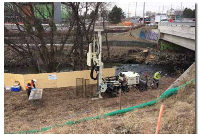
A Landshark Drilling field team works on an environmental investigation which required the installation of multiple monitoring wells along a sensitive watershed.
