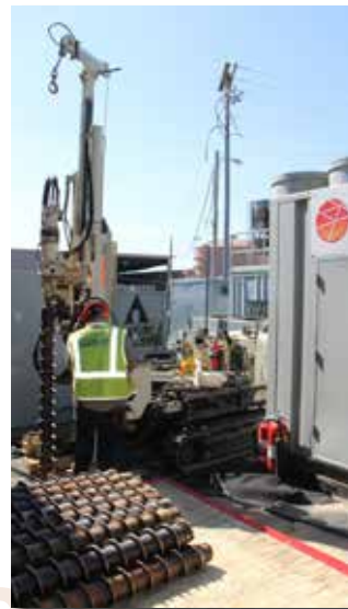
(above and below) Drew Small with TRS contacted Geo Lab to assist with ERH electrode installation at an active manufacturing facility near Murphy, NC. For this most recent phase, Geo Lab installed supplemental electrodes, as well as obtained continuous soil samples with soil temperatures around 200 degrees F. A 7822DT pulled the continuous hot soil samples, from 100 ft. bgs, by advancing a Macro-Core® sampler with stainless steel liners to withstand the heat. Following the sampling, Geo Lab installed multiple electrodes to greater than 100 ft. using hollow stem augers, requiring very careful handling of the steaming mud. After completion, Drew Small said that in the early stages of the project he had his doubts as to whether the scope of work could be completed. "I was impressed with the capability of the rig and your guys during this install," he said. "I wasn't sure it was possible."
