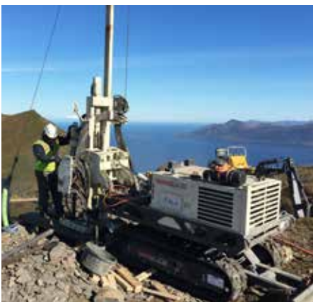
Darrin VanDehey, Driller, uses air rotary with a 6712DT.
