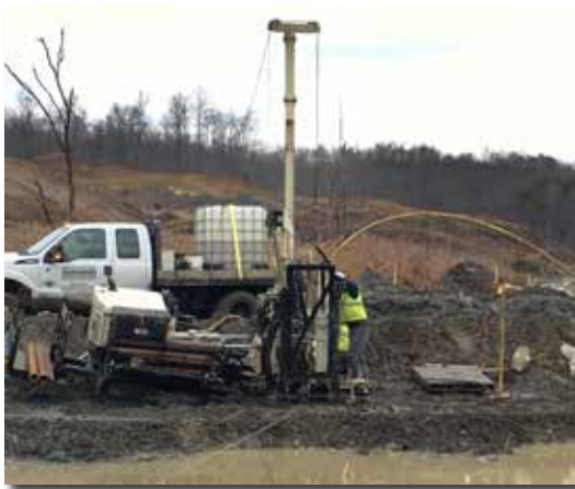
(above & below) Because temporary 'roads' were uneven, oscillating the 3230DT and 7822DT drill masts made adjusting to side-hill terrain easy.
