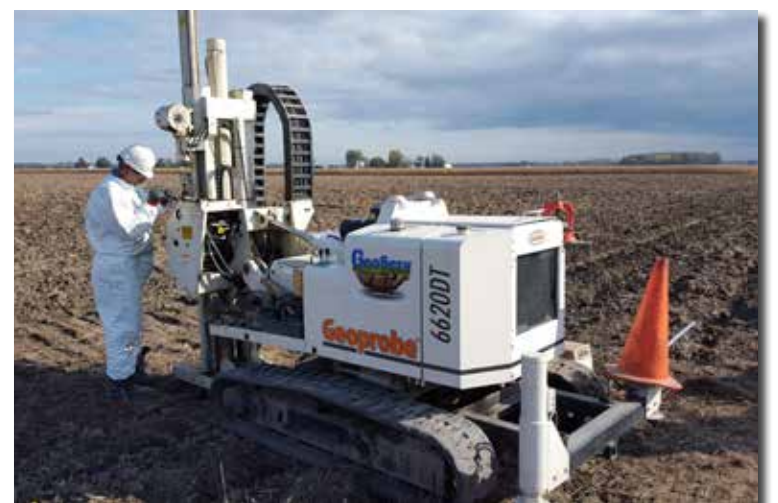
Because of the expanding clay in the formation, Robert Hansen, GeoServ Driller, sometimes recovered a 5-ft. soil core with only a 2.5-ft. push.
