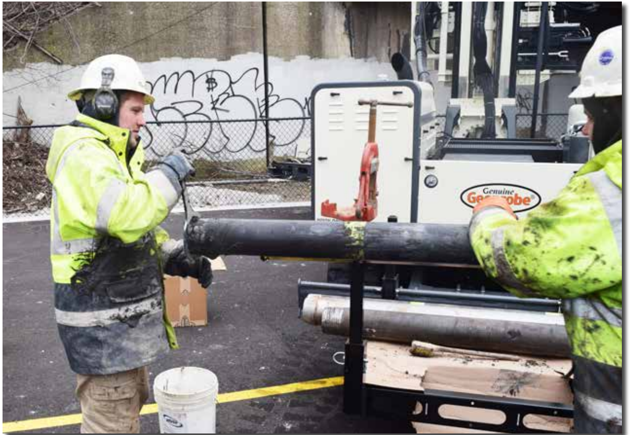
Adam Sweet, (left) Vice President of Horizon Construction and Exploration, and Robert Albinger recover 6-in. samples with the 3230DT on its first project in Milwaukee, WI.
