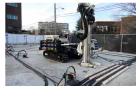
(above and right) Soil confirmation borings had previously been completed on this Electrical Resistance Heating (ERS) site in downtown Seattle, WA. Holocene Drilling returned with their new 7822DT to confirm the project's success. The small footprint of the 7822DT allowed the company to access the boring locations within a very confined area.
