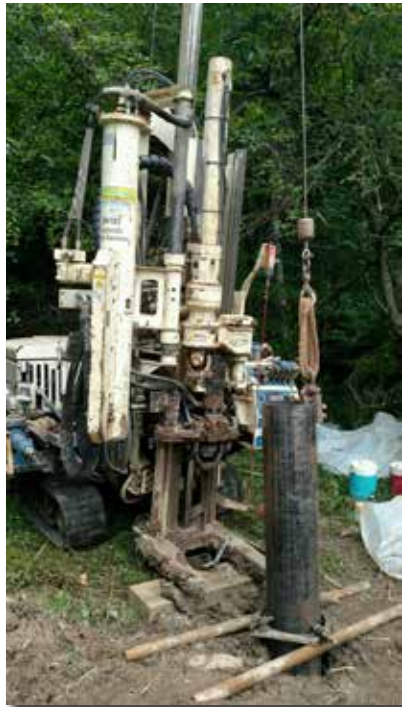
Installing 10-in. steel casing with the 7822DT.
