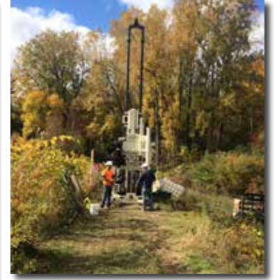
Derek Fennell and Bob Gannon complete split spoon, Macro-Core® soil sampling, and wireline rock coring on an earthen dam.
