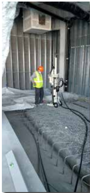
Drew Gagnier, with Trinity Drilling, uses a 420M to complete a soil investigation inside Sunnyvale, CA, Google complex.
