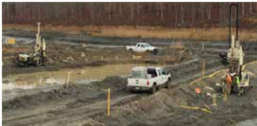
(above & below) Because temporary 'roads' were uneven, oscillating the 3230DT and 7822DT drill masts made adjusting to side-hill terrain easy.
