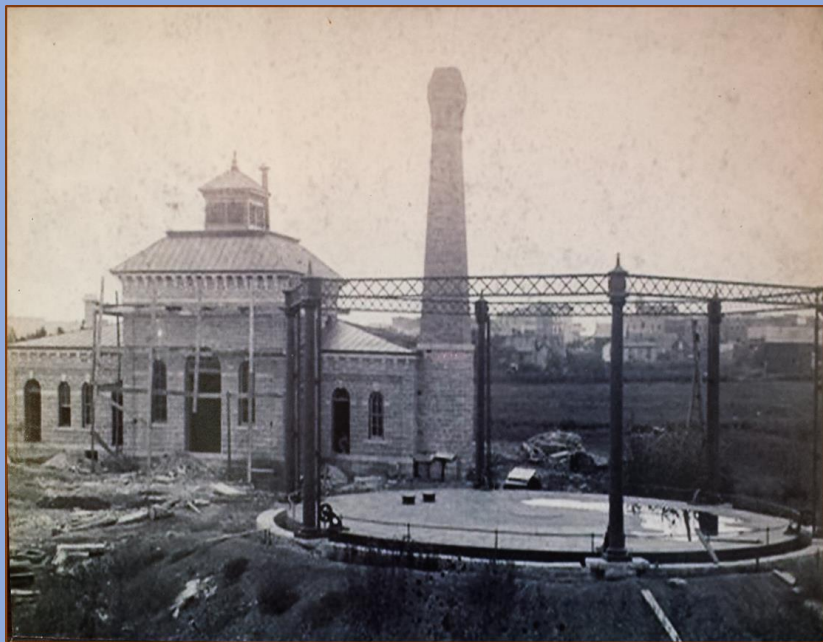
The Wellington, KS Manufactured Gas Plant (MGP) under construction (circa 1886) gas holder in foreground
