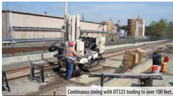
Continuous coring with DT325 tooling to over 100 feet.
