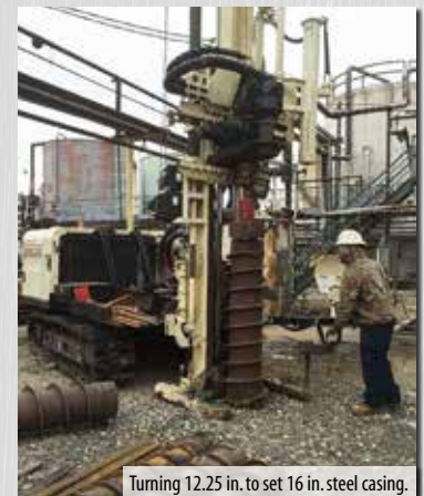
Turning 12.25 in. to set 16 in. steel casing.
