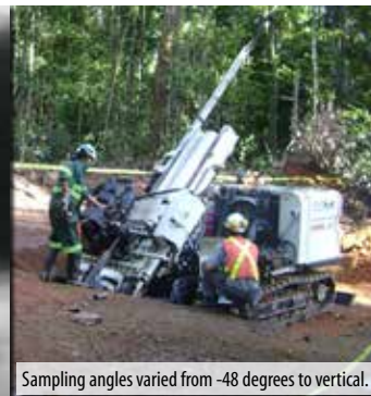
Continuous coring with DT325 tooling to over 100 feet.
