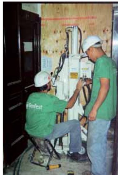
The GeoTest team operates a 420M in the building's basement to obtain geotechnical samples as part of the structural design requirements for a new elevator shaft.
