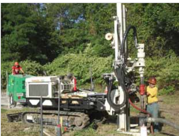
Michael Jordan, Rig Operator for Stone Environmental, uses a downhole air hammer with a 7822DT. Over 160 multi-function wells were installed at the site in four weeks.
