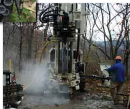
(left and below) EnviroProbe used a 6-in. downhole (DTH) hammer with an 8-in. bit and API IF rods to install the cased monitoring well. Dale Kestner, Driller for EnviroProbe, is at the controls of the 8040DT.
