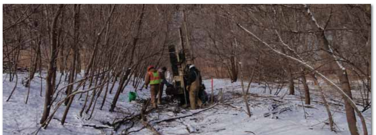
(below and lower right) Thiele Geotech uses their 6620DT to retrieve soil samples at the former Ash Lagoons near Omaha, NE. Redevelopment construction of the area will involve the excavation and disposal of approximately 8,200 cubic yards of soil. The field team members were Cory Bachman, Driller; James Beutler, Driller’s Assistant; and Dennis Anderson, Senior Geologist.
