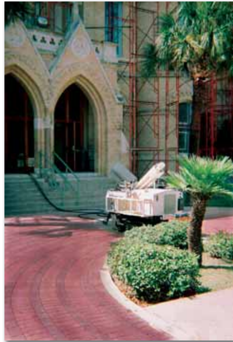
A Geoprobe® 54LT served as an outside power source while the GeoTest Services field team collected soil samples with a 420M inside the building.
