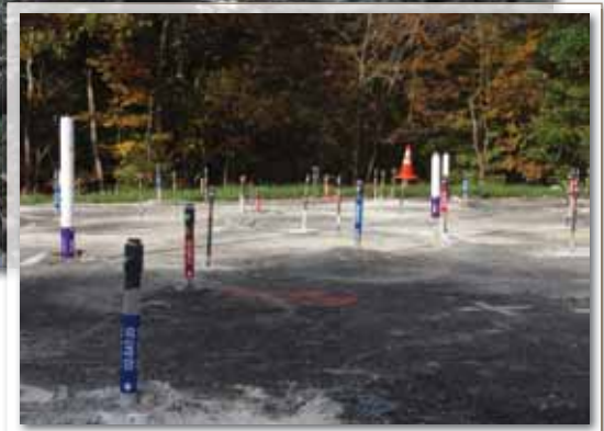
(inset) Just a few of the 160 multi-function wells installed at the site. (above) Matthew Muir, Rig Operator for Stone Environmental, uses 3.25 in. casing to collect soil samples at a former drum burial site in New England.
