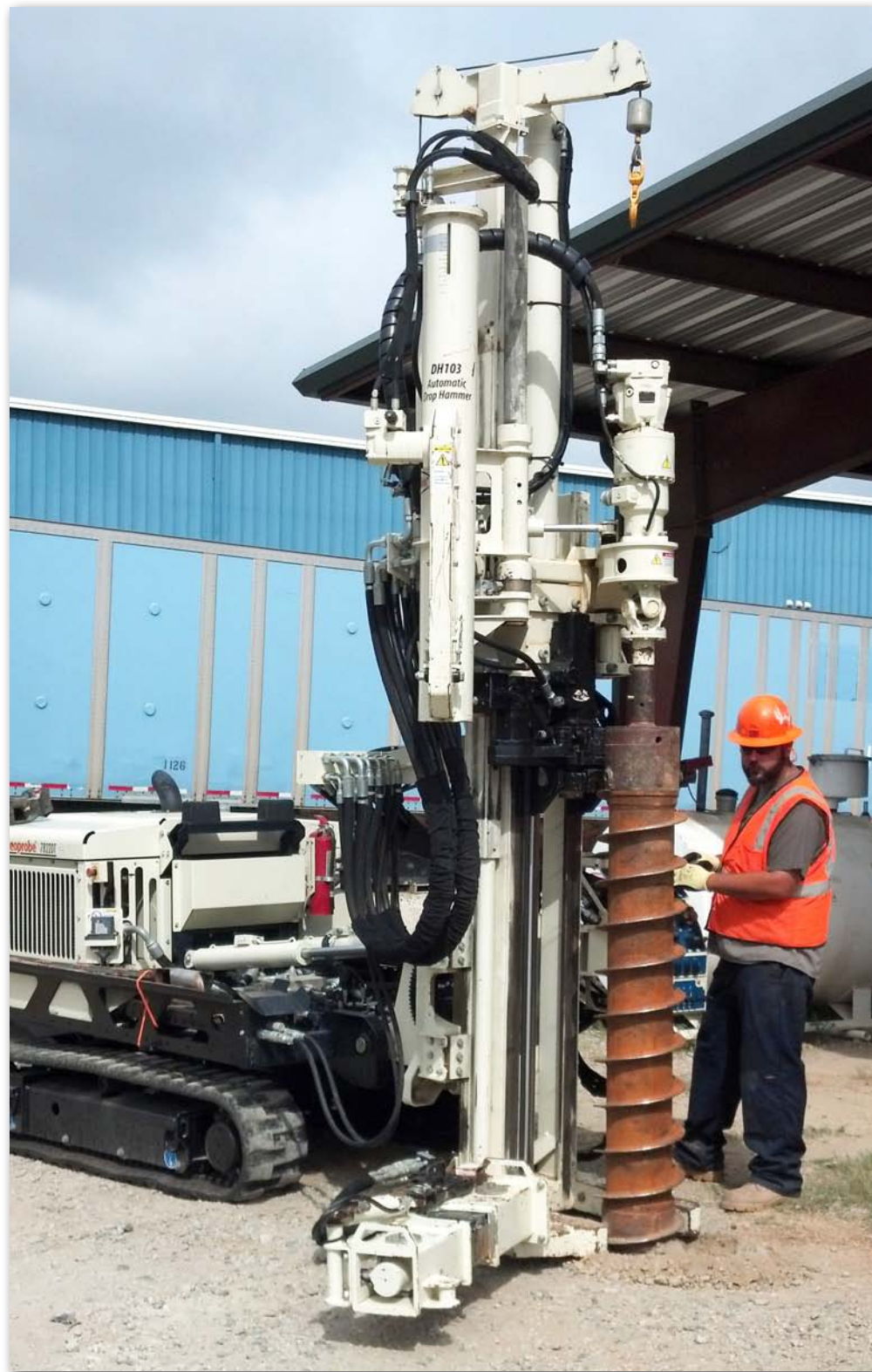
Phillip Ricker, Geo Lab Lead Driller, advances 8.25 in. ID hollow stem augers with their 7822DT for 4-in. PVC recovery well installation.
