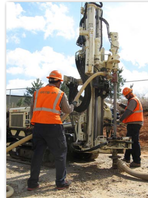
Robert Taylor and Phillip Ricker set up to bore through rock with the Geo Lab's 7822DT and 3.5 in. DTH Air Hammer.
