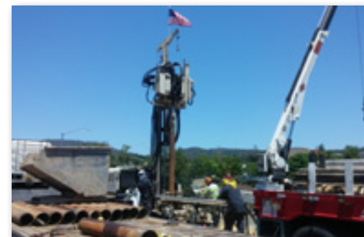
8140LS Sonic owned by Cascade Drilling, LP,
