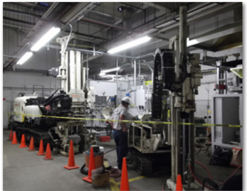
A Vironex Field Team, Mike Haske and Robert Lopez, use a Geoprobe® 8040DT and 6610DT at an industrial facility in Los Angeles, CA, for direct push injection of calcium polysulfide for hexavalent chromium (Cr(VI)) treatment. The 6610DT (foreground) was injecting in the shallow treatment intervals (50 ft.) while the 8040DT was injecting into the deep treatment intervals (80 ft.).
