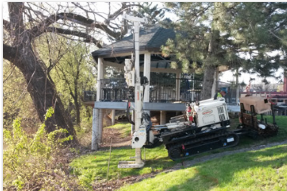
According to Tom Ulrich, Driller for Stearns Drilling, the articulating derrick of the 7822DT was very helpful when positioning the rig for sampling on the steep river banks. The pavillion shown in the background provides outdoor seating for the Gas House Restaurant.
