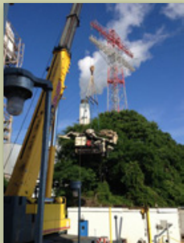
This project involved the installation of five 4.0 in. dual phase recovery wells set adjacent to a sea wall which required the use of a 300-ton crane to lift and position the 8140LS sonic rig. A network of aboveground gas pipelines had to be cleared which dictated the need for the crane lift.
