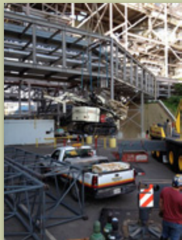
This project involved the installation of five 4.0 in. dual phase recovery wells set adjacent to a sea wall which required the use of a 300-ton crane to lift and position the 8140LS sonic rig. A network of aboveground gas pipelines had to be cleared which dictated the need for the crane lift.
