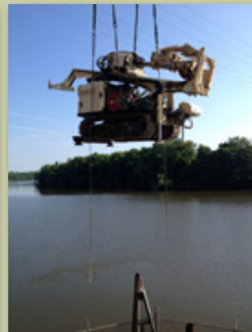
This project involved the installation of five 4.0 in. dual phase recovery wells set adjacent to a sea wall which required the use of a 300-ton crane to lift and position the 8140LS sonic rig. A network of aboveground gas pipelines had to be cleared which dictated the need for the crane lift.
