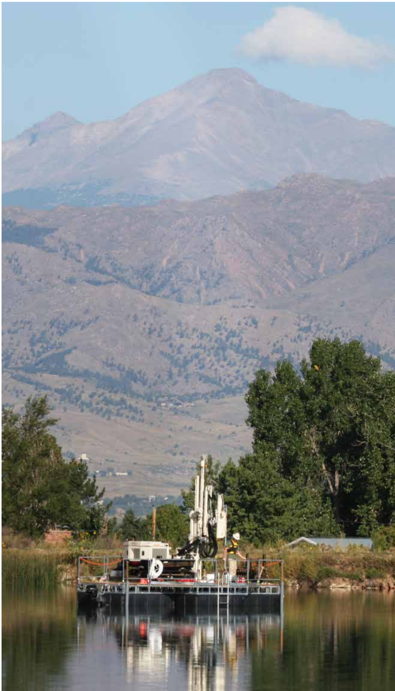
A total of three holes were drilled to approximately 40-50 feet below the water surface into the underlying bedrock to collect soil and bedrock samples.
