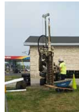
AJ Benjamin, EPI's 7822DT Operator, uses the machine to turn 6-5/8-in. augers.
