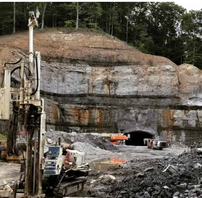
Geotechnical drilling for a future HDD pipeline boring using 3.25-inch augers and NQ coring in West Virginia (top left). Mineral exploration sampling using 5-foot split spoons with DT45 for casing down to 110 feet in Illinois (top right). Geotechnical structure borings for a new coal mine belt line using 3.25-inch augers and NQ coring in Eastern Kentucky (bottom left). DT35 sampling with 4.25-inch augers setting 2-inch monitoring wells in Cincinnati (bottom right).
