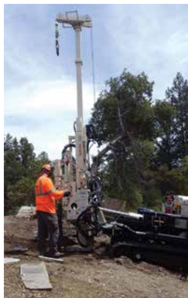
Geoprobe® 7822DT rotary wash drilling to 150 feet with 4.75-inch tri-cone (left). Exploration on top of fill edge with hollow stem, auto drop hammer, modified California samples and direct push Macro-Core® sampling to determine fill/native and native/sedimentary formation contacts (center). 7822DT hollow stem exploration for proposed sidewalks and road shoulder investigation on steep bank (right).
