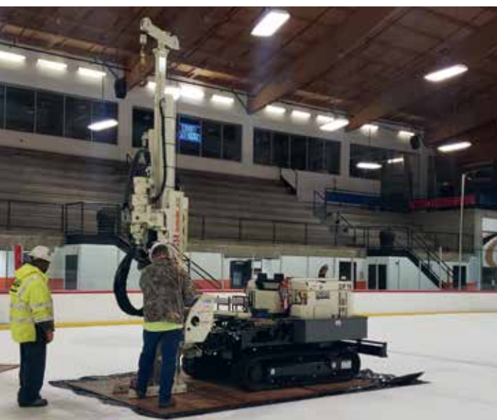
Gregg Drilling LLC conducts Macro-Core® sampling at the former Anaheim Ducks practice facility (left). They chose the Geoprobe® 7822DT for its narrow width, low track load on the ice surface (4.6 lb./in 2 ), rubber tracks, and ease of operation with the wireless remote. The fact that it was only three months old was also an advantage, keeping dirt from falling off the tracks onto the rink (right).
